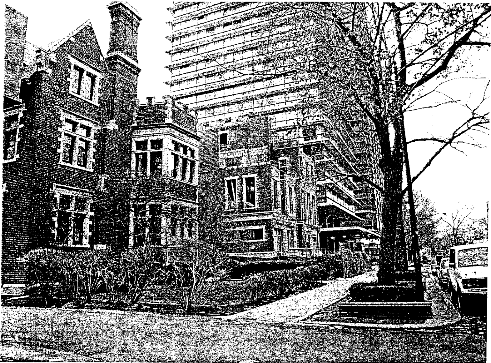
Figure 5. View of Oakdale. Meeberville Historic District Cook County, IL.
